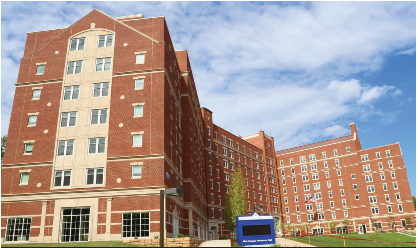
The new Mid-Campus Residence Hall on Harold Lewis Drive and Ella Grasso Boulevard opened with the 2015-16 academic year.
